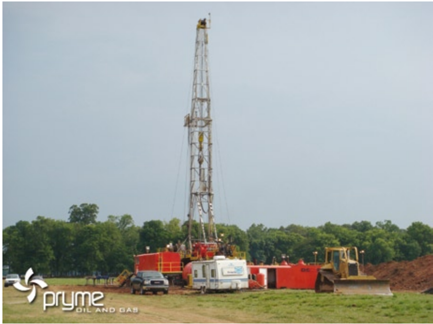
Drilling continues in Turner Bayou
