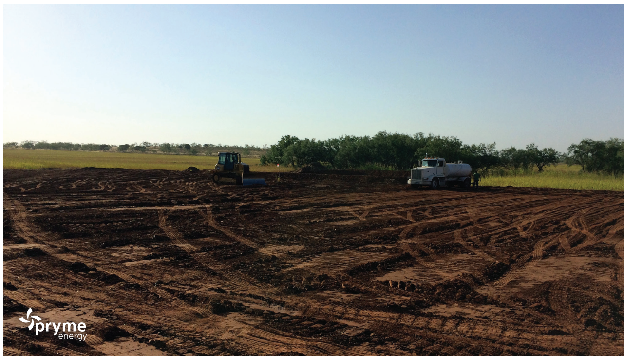
Site preparation on the Hopes-Boles PU #1 well
