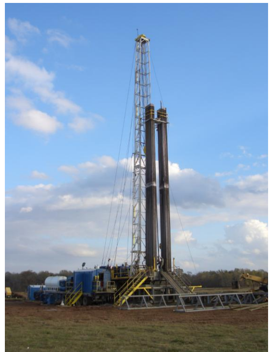
Drilling of Bordelon 25 No.1 in Turner Bayou
