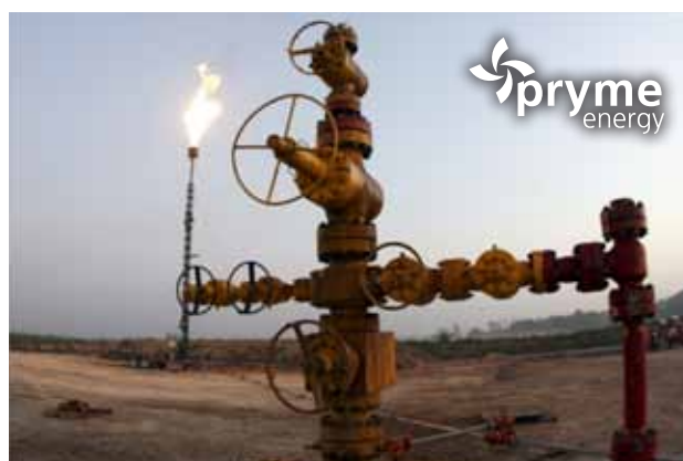
Flow testing the Deshotels 13H No.1 well in the Turner Bayou Chalk project
