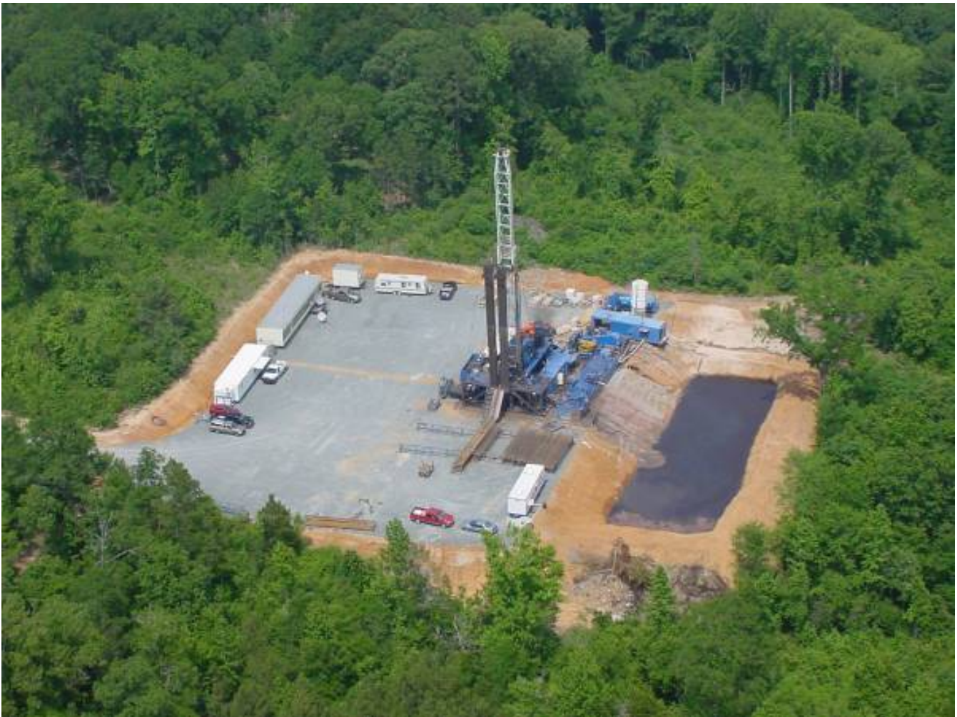
Drilling of the Patterson 16 No.1 in the Raven Project
