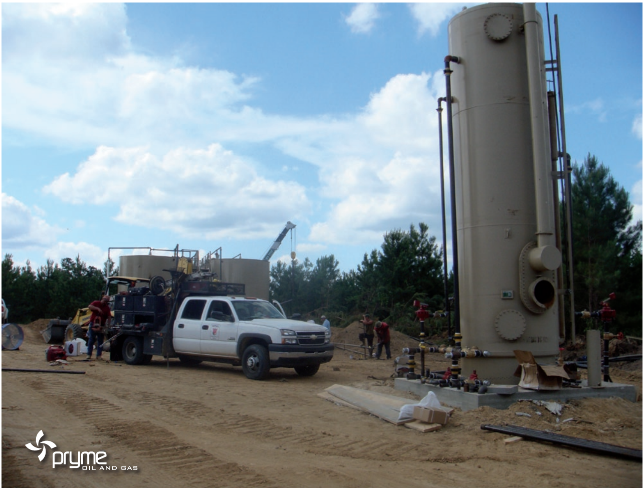
Installation of production facilities at Crosby 16 No.1, Kelly Hill Prospect
