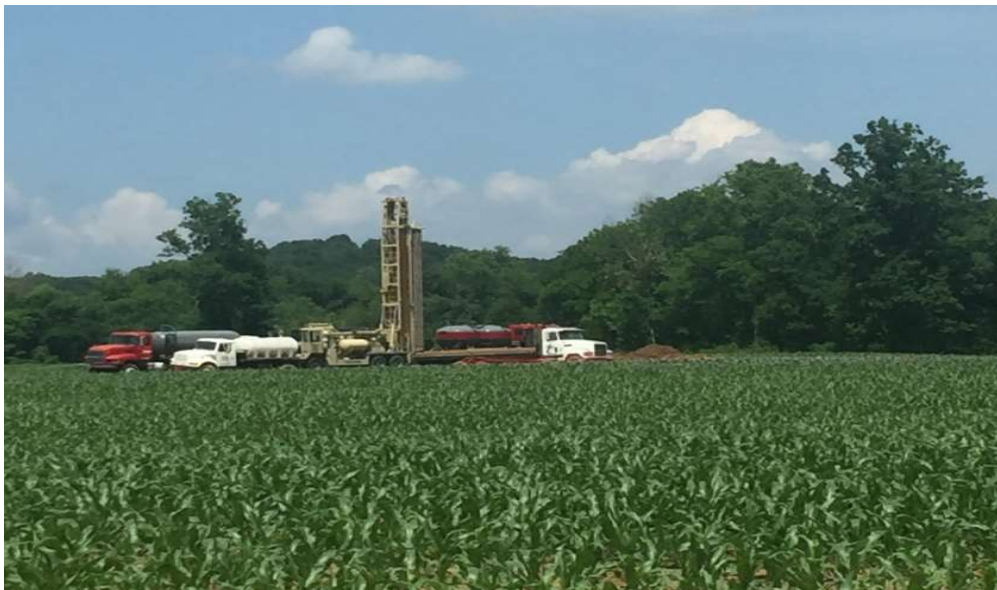
Drilling the Weldon Young #1A well in Kentucky.
