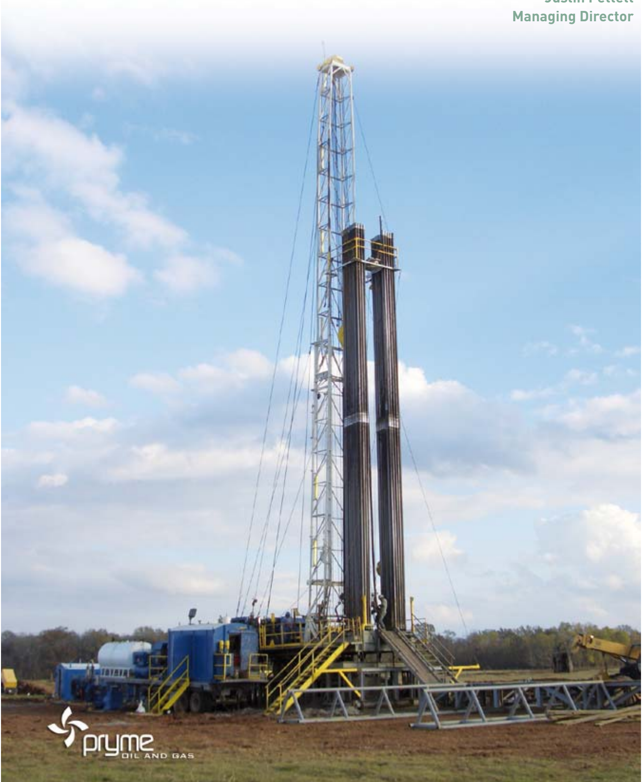
Drilling of Bordelon 25 No.1 in Turner Bayou
