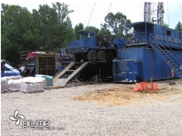
Drill rig on the Spinks Middlebrooks 11-1 well in Raven
