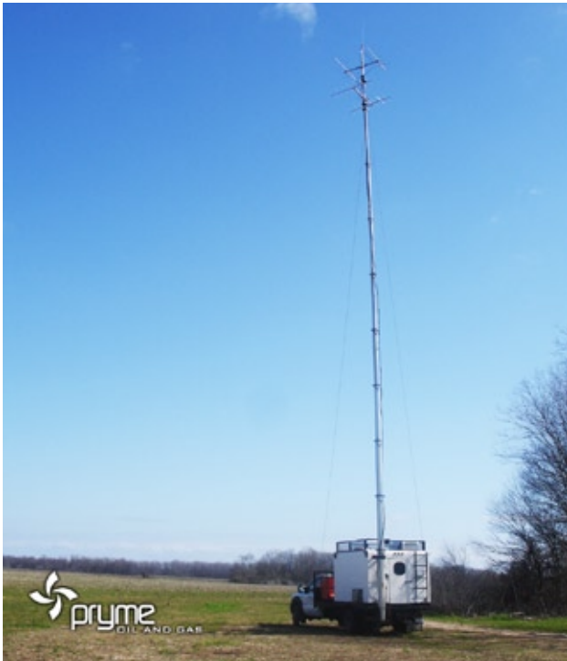
Seismic data wireless receiving tower in the Turner Bayou Field
