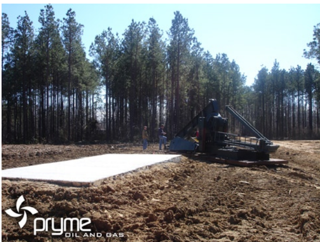
Completion of the NWR No.16 - pump jack and pad
